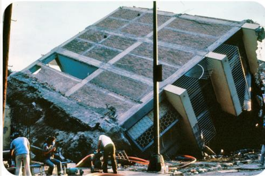
Liquefaction of sediments in Mexico City caused the collapse of many buildings in the 1985 earthquake. M 8.0
