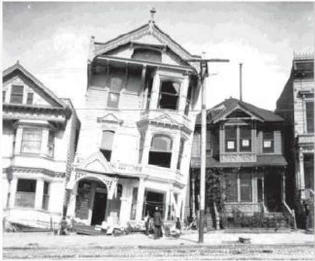
Houses damaged by the 1906 San Francisco Earthquake M 7.9
