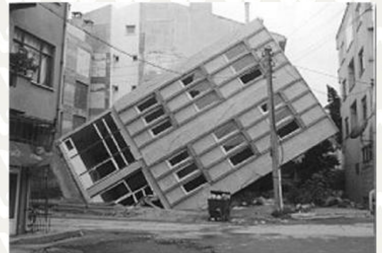
Rotation and settlement of building due to liquefaction, Turkey, 2001 M 7.4
