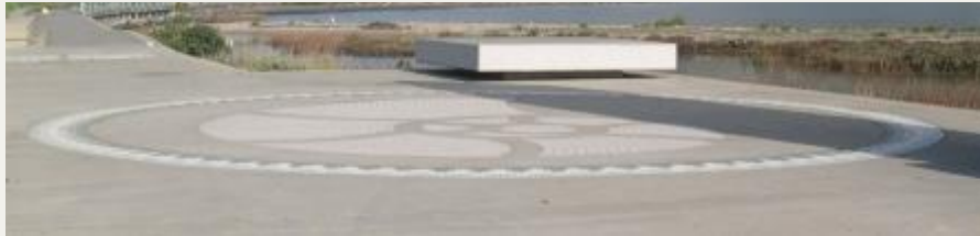
Pump Station – Detail/closeup of a particular feature
