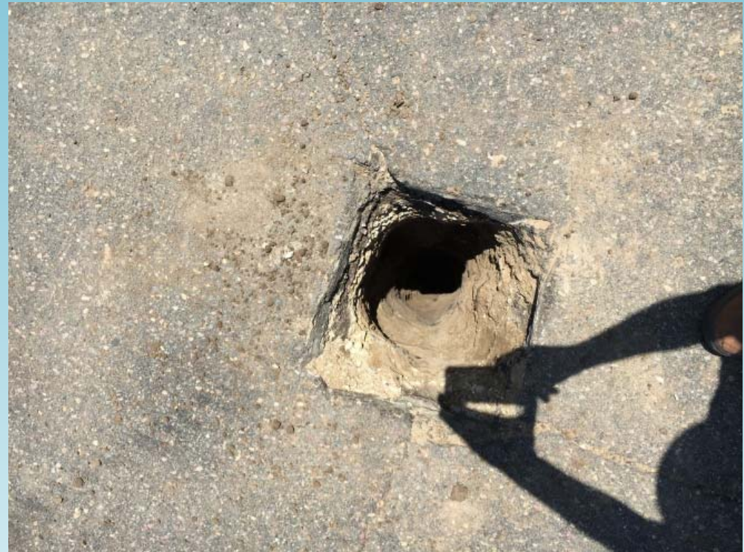
Excavated Hole (to pipe bedding)
