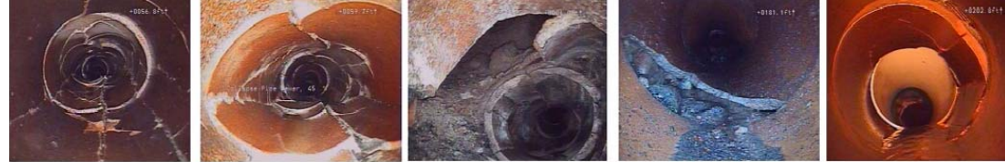
Sample video images of sewer lines showing broke pipe, partial collapses, offset joints & intruding laterals.
