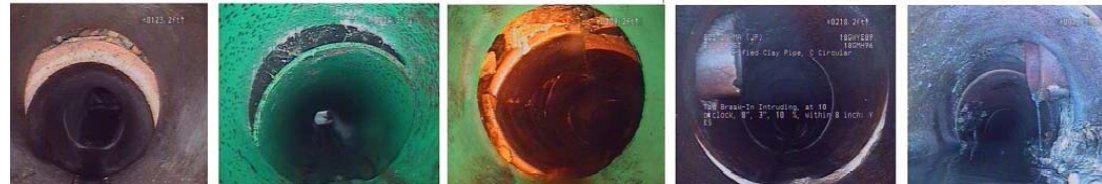
Sample video images of sewer lines showing broke pipe, partial collapses, offset joints & intruding laterals.
